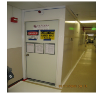
Rigid containment barrier
