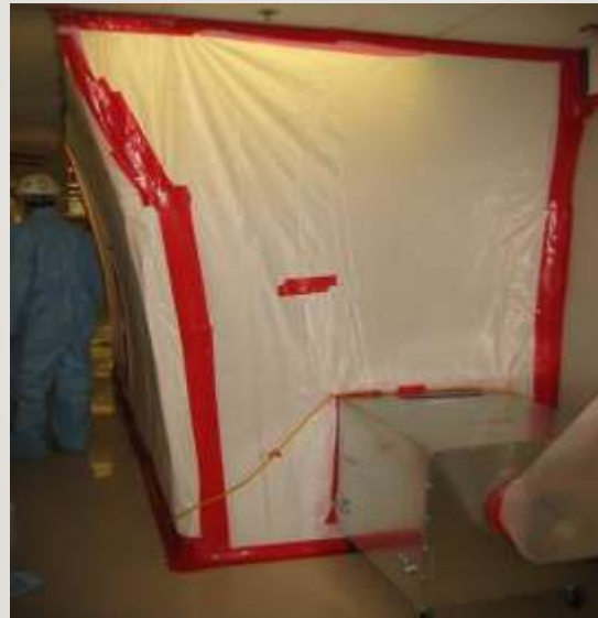
Non-rigid containment barrier
